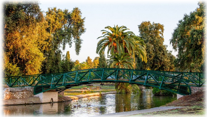
Mooney Grove Bridge Renovation
